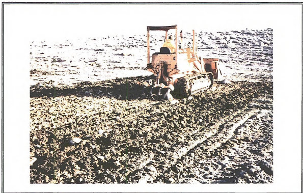
Photo 10: Ripping biosolids into the soil
